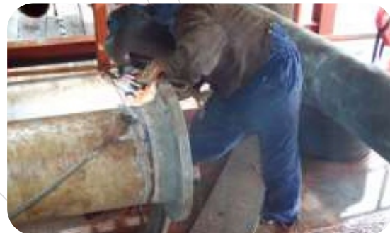
Welding in Progress (Tie in Joints)
