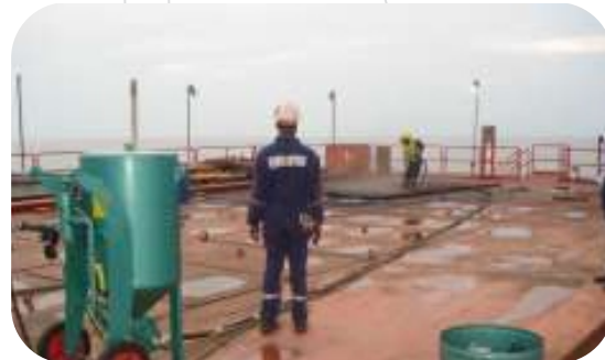
Grit Blasting of Floor Plates
