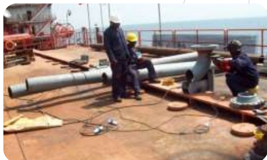
Fabrication of Pipes, Flanges and Elbows
