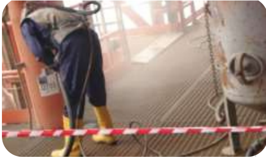
Grit Blasting of Floor Plates
